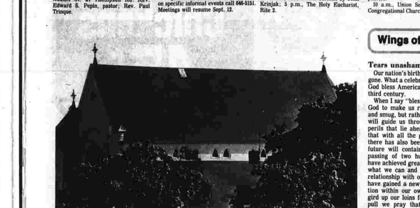
Roofline of St. James Church
